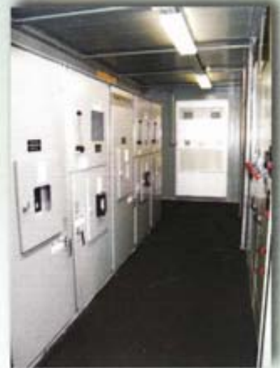
Outdoor Walk-In Metal Clad Switchgear
