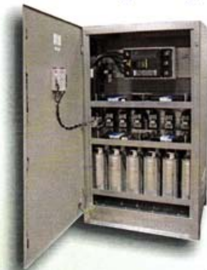
Figure 2 : Power Factor Improvement (PFI) Plant
